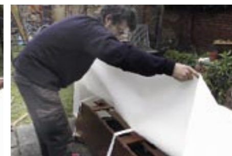
12 The cover was fully put on, again with more silicone in way of staple runs. We were racing the rain at this point!
