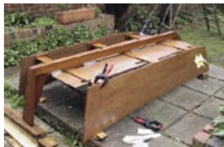
8 Ready for the covering. It's important to set her up right for this: note blocks, and two of 20 clamps (overnight from Screwfix).
